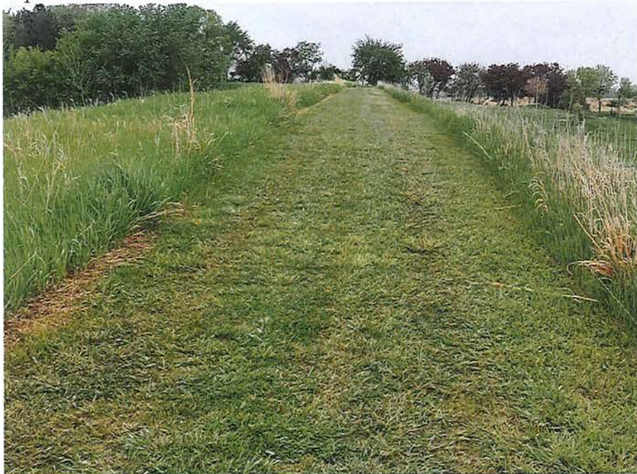
Crest of Dam
