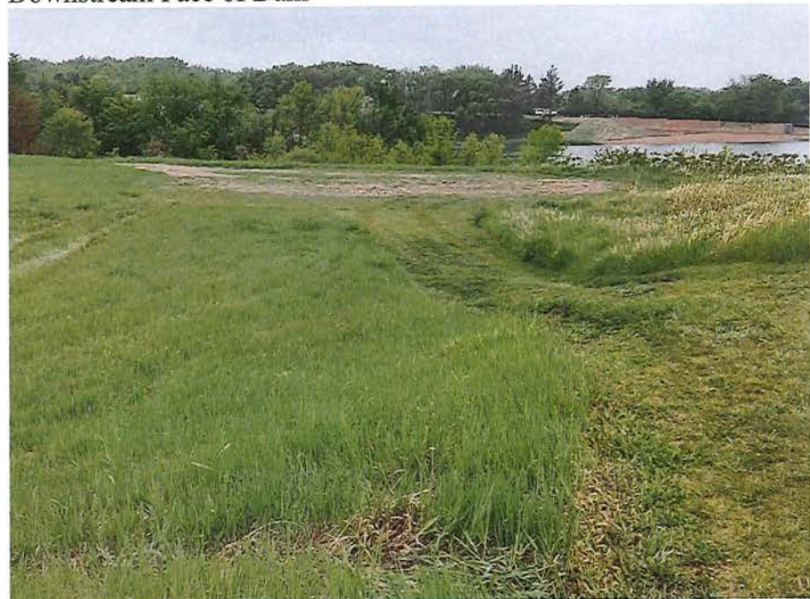
Emergency Spillway (Looking SW)
