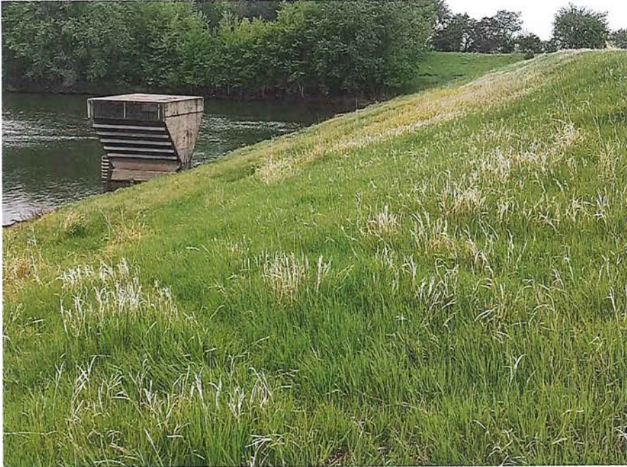
Upstream Face of Dam
