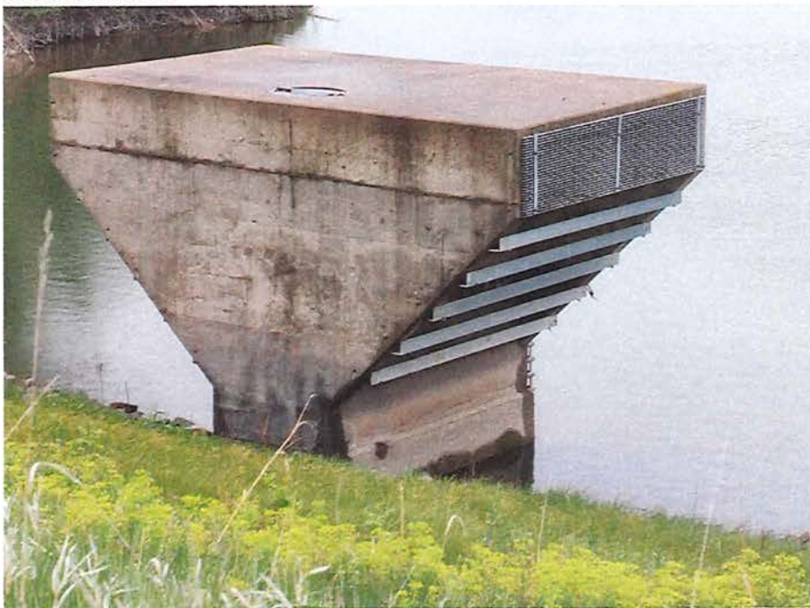
Riser Structure – Right View
