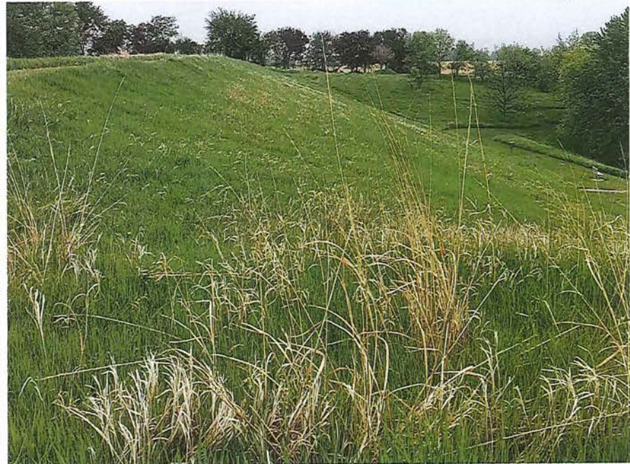
Downstream Face of Dam
