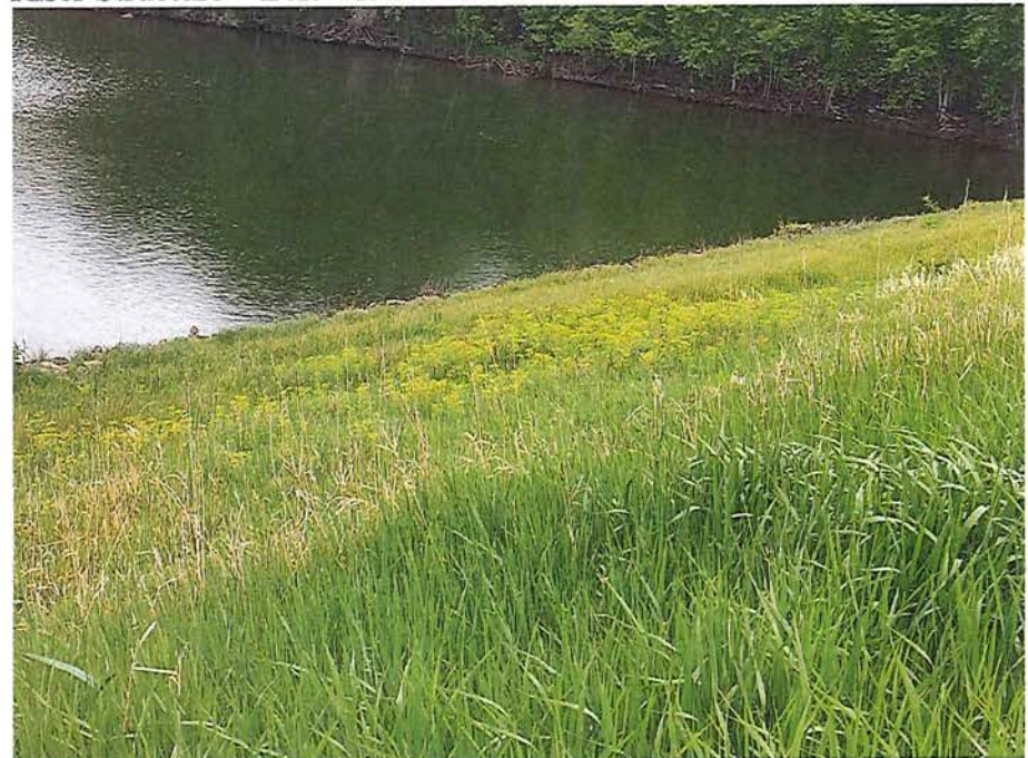
Leafy Spurge on Upstream Face of Dam Embankment
