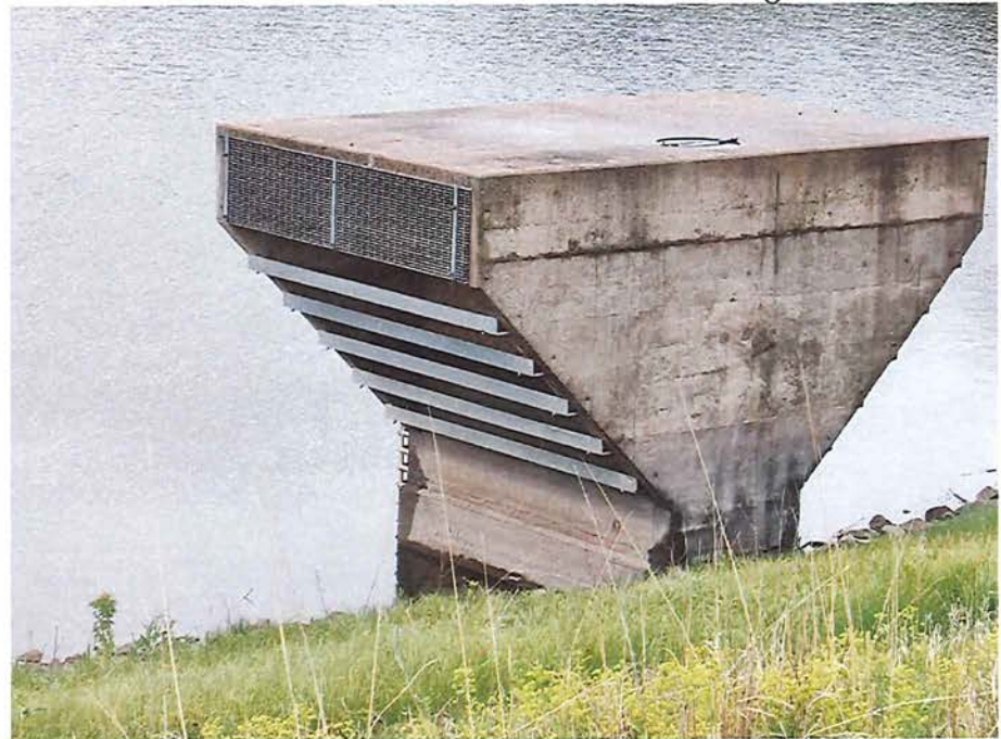
Riser Structure – Left View
