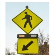
Rectangular Rapid Flashing Beacon
