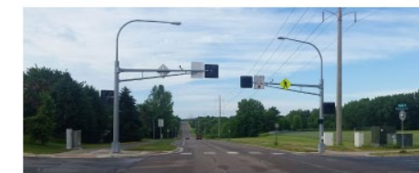
High-Intensity Activated Crosswalk Beacon
