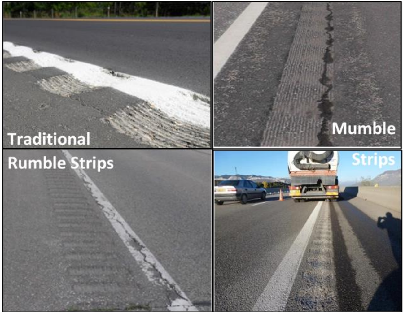
Figure 3-5. Mumble Strip Design – Traditional versus Mumble Strips Wave-shaped design produced less external noise than MnDOT's current design
