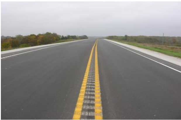
Centerline Rumble Strips
