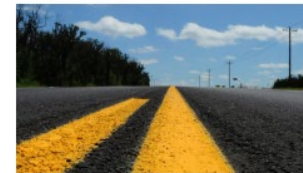
Typical Seal Coat (Chip Seal)
