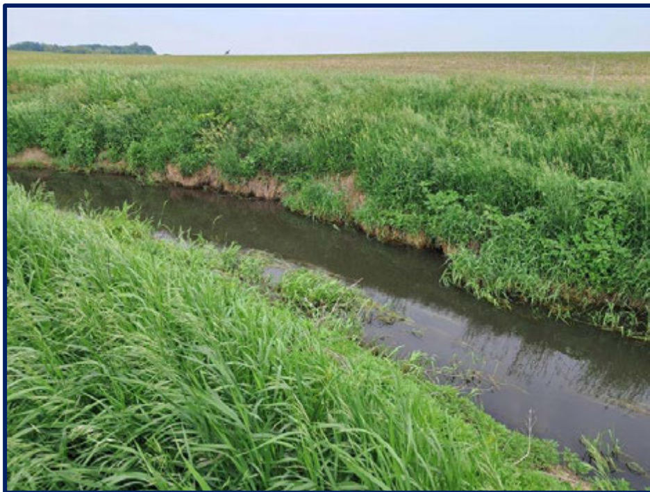
Figure 3. CD 12 Open Ditch Downstream of CD 20 Mainline tile outlet
