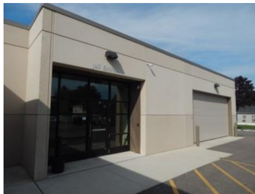
(Main Entrance to the Redwood County Jail)
