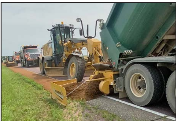
Redwood County Highway Department crews re-gravelling shoulders in August 2021
