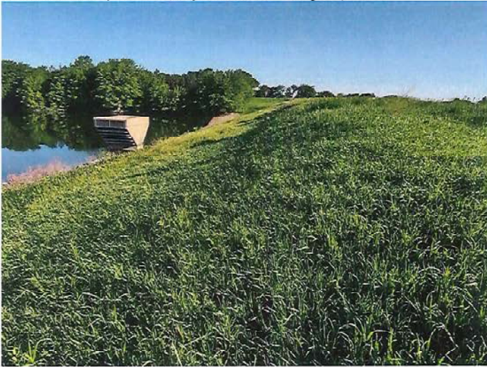
Upstream Face of Dam
