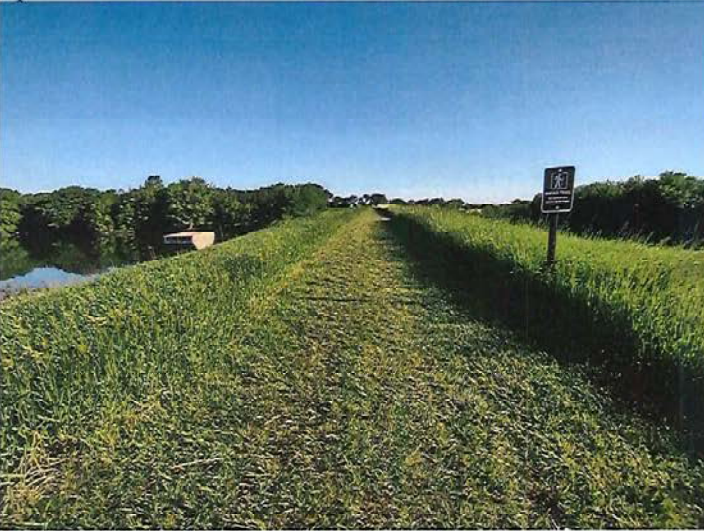
Crest of Dam
