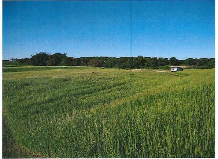
Emergency Spillway (Looking SE)
