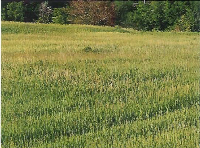
Small tree/bush growing in the Emergency Spillway to be removed.
