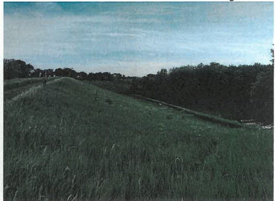
Downstream Face of Dam
