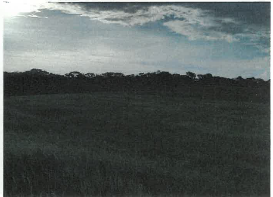
Emergency Spillway (Looking SE)
