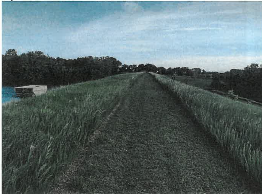
Crest of Dam
